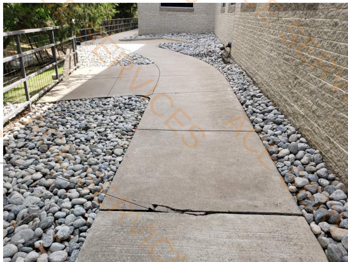
4 5900 NORTH SIDEWALK DEMO
