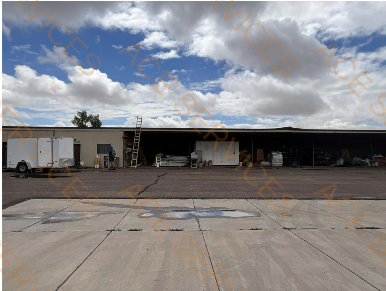
NORTH ELEVATION OF VEHICLE STORAGE BUILDING
